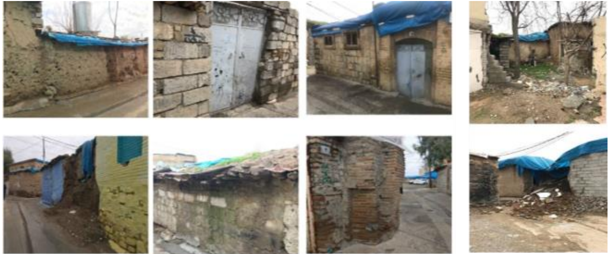
Figure 3: buiding materials and various oblesence observed in the area (By researcher).
